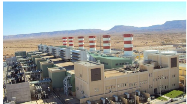
Figure 1. Western Mountain Gas Power Plant, Nalut, Libya
